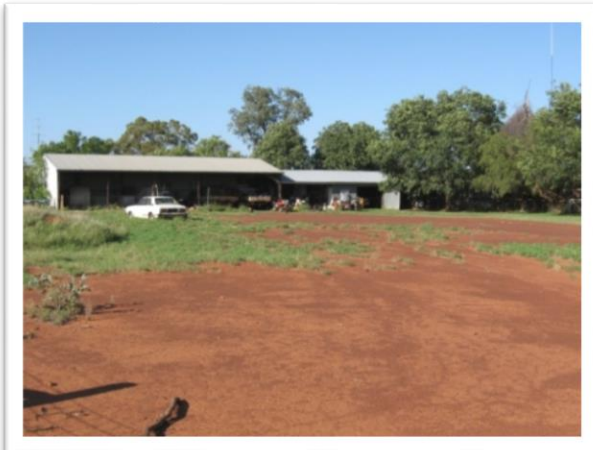
Workshop and machinery shed – Kandimulla
